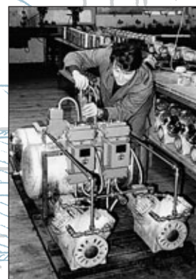
Compressor unit being assembled (1968)
